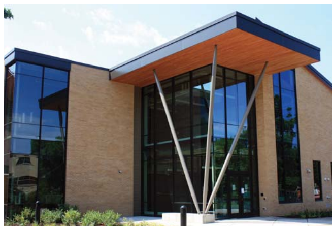
Edgewood's new Visual and Theater Arts Center, The Stream
