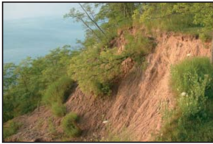
Erosion eats away at CUW's shoreline.
